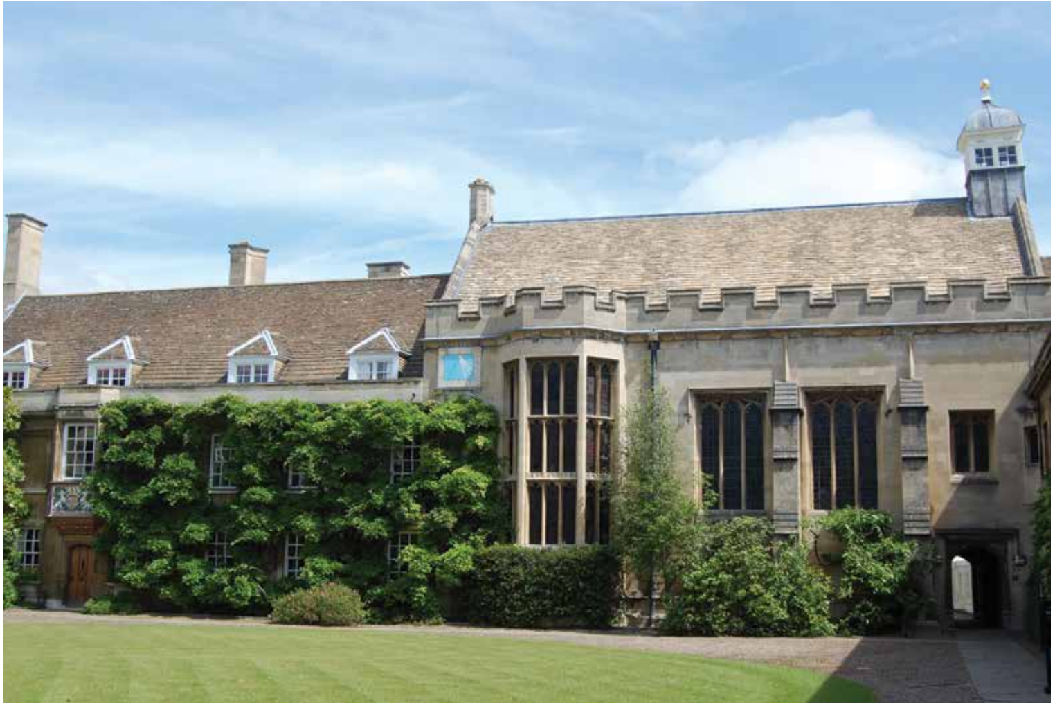
The Hall looks stunning with its new roof.
