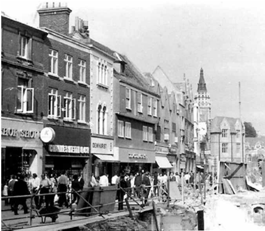
Demolition of half of Petty Cury
