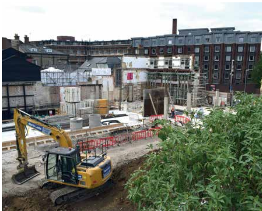
King Street Development in progress, September 2021
