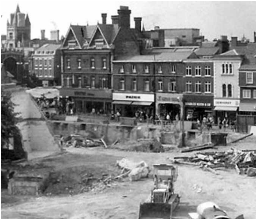
Extent of demolition of Petty Cury
