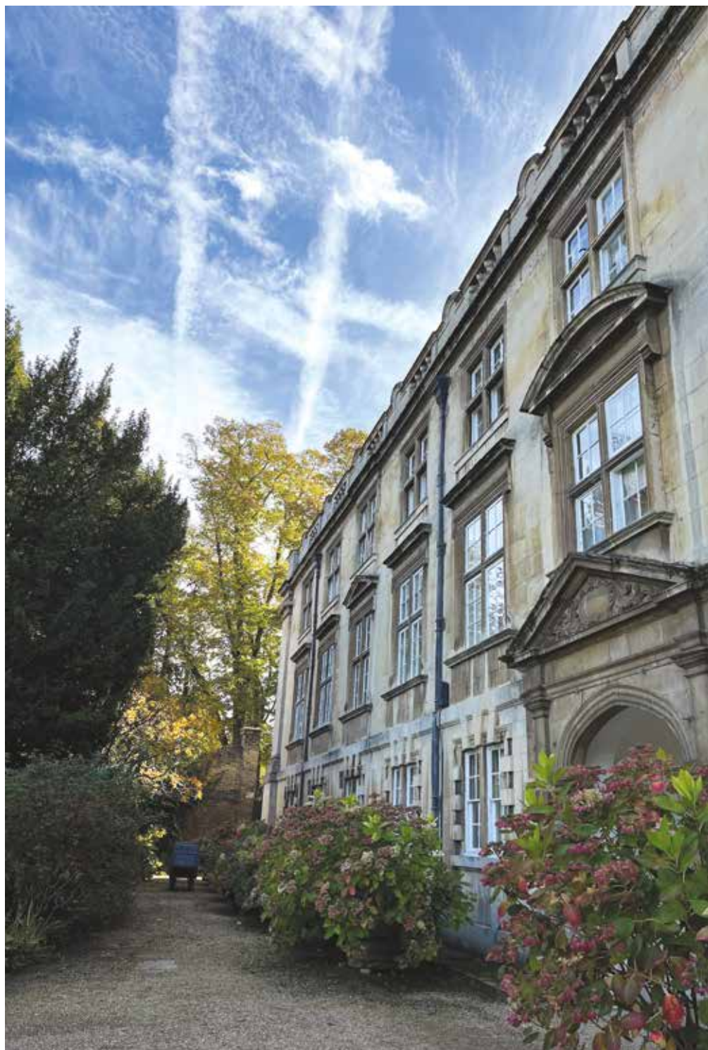
The Fellows' Building
